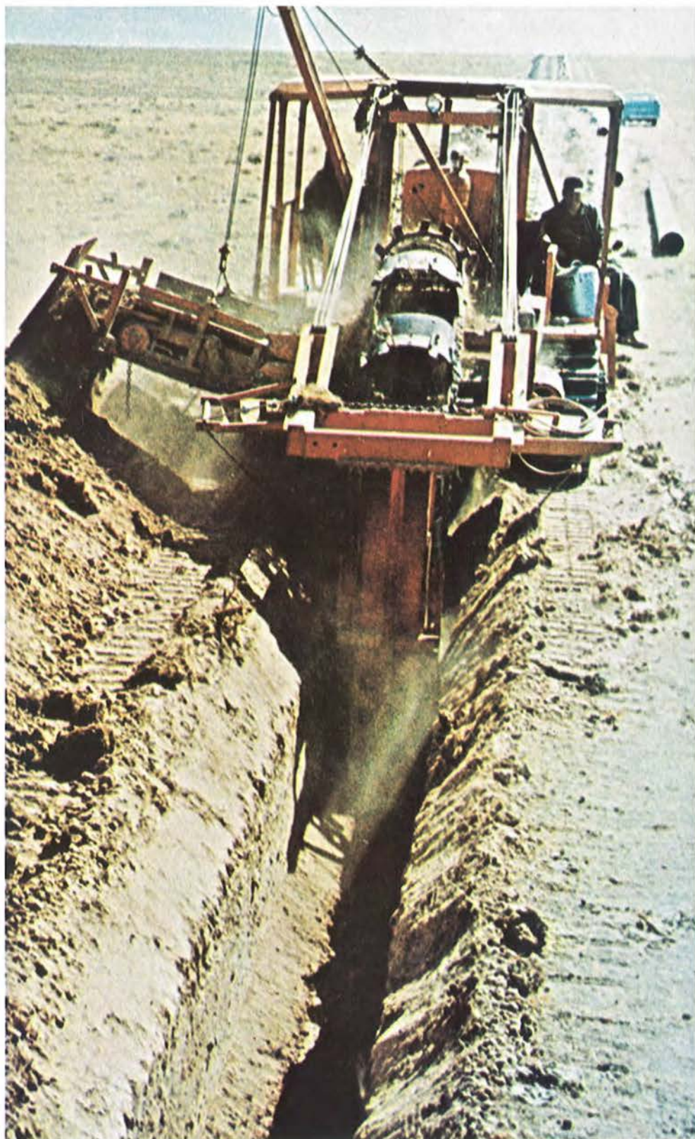
The trench for the gasline is dug with a backhoe or a trenching machine.
