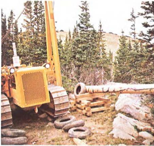
To protect alpine and other fragile areas from "cat tracks," old tires and boards were used to cushion ground vegetation and soils.
