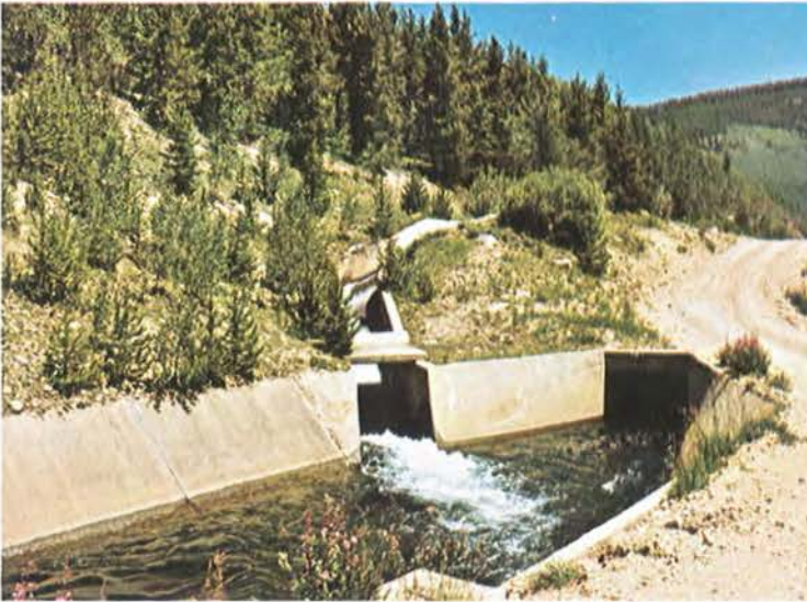
Open drop structure.
