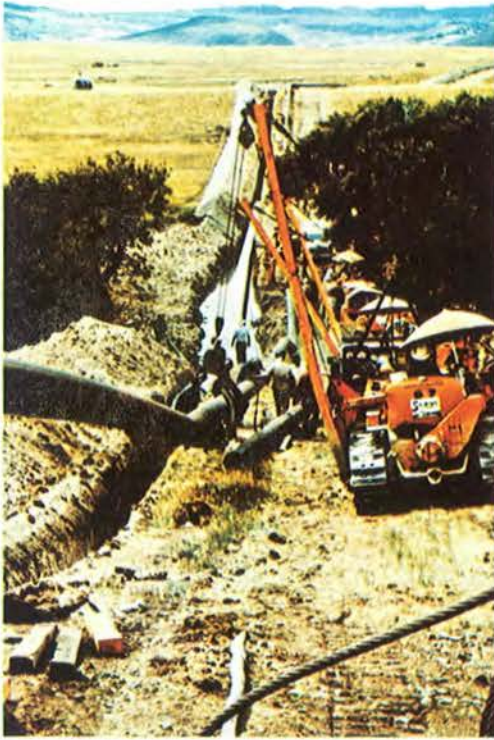
Above A 16" gasline crosses a small stream. Note the 30' gap in the trees and the extra width of the trench at the stream.
