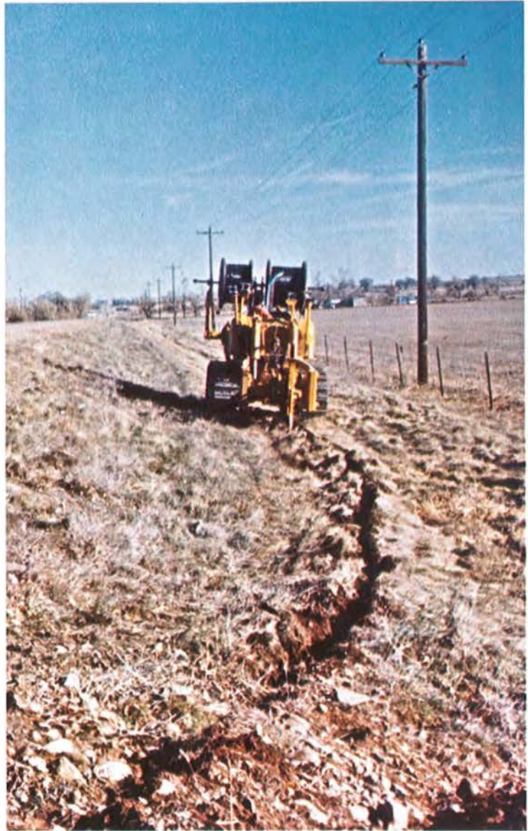
This telephone cable is being installed by a vibrating plowshare drawn by a tractor that also carries its own supply of cable.
