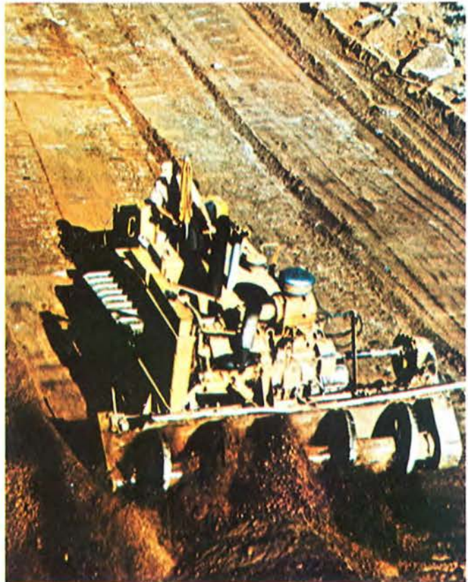
Above right A 20" pipe is being installed. Note the concrete weight at the stream crossing. This weight holds the pipe in place (prevents floating) and protects the wrapping from water, ice, and gravel scouring.
