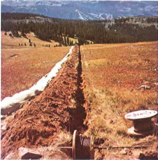
The backhoe then dug the rest of the ditch. The pipe was welded together off the tundra. A winch at the upper end of the ditch pulled the pipe into place.
