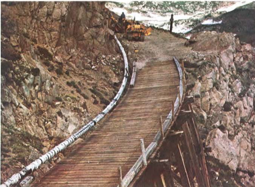
Visual impact was minimized in this difficult situation by burying the gas line in the roadbed and supporting it across this old railroad trestle.
