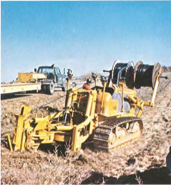
This telephone cable is passing into the feed chute of a vibrating plowshare being drawn by a tractor.
