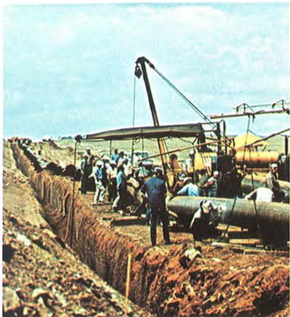
Several welders may work simultaneously on a large pipe.
