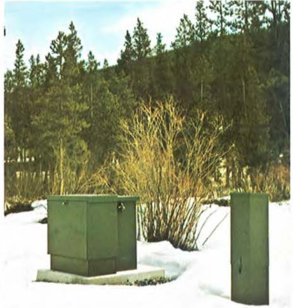
Aboveground facilities such as this padmount transformer and secondary pedestal are necessary, even for underground systems.
