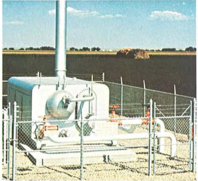
This "heater-separator" unit is on a gas well in irrigated farmland.
