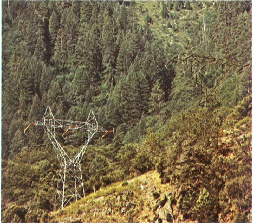
Two similar towers—except for color. The upper tower has been painted dark olive.
