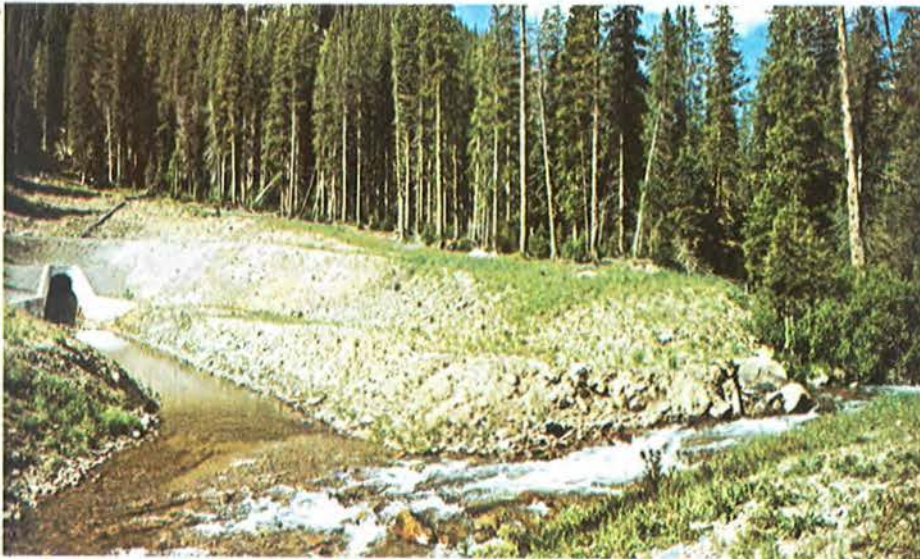
Other components of the water collection system are tunnels, gauging stations, weirs, and energy dissipaters.
