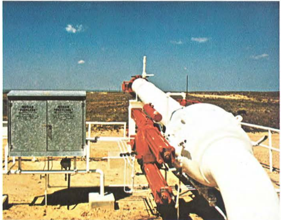
Automatic controls for this sphere launcher are in the metal "doghouse." The unit drops spheres into the gasline to aid in removing liquids from the gas. Such units are used primarily in gathering systems.
