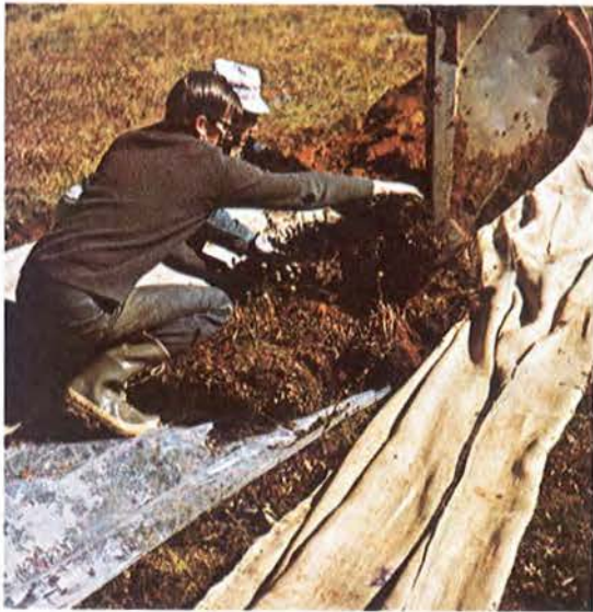
The top layer of tundra was excavated with a specially designed blade, placed on plastic by hand, covered with burlap, and watered.
