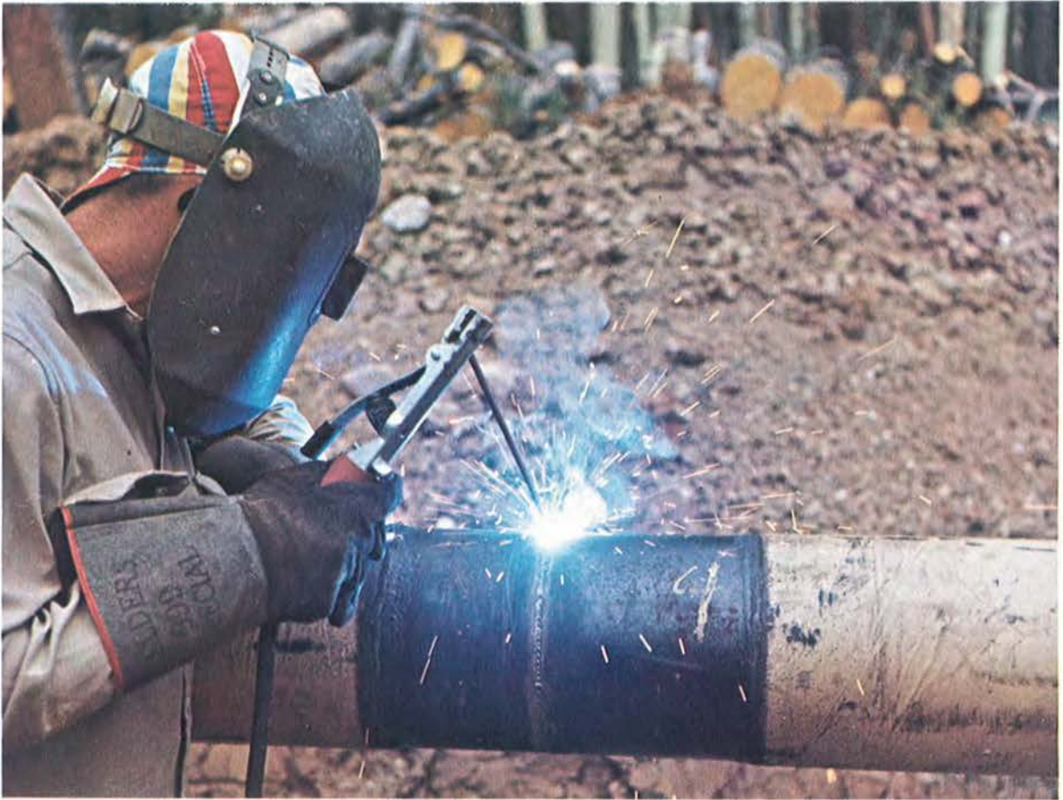
After the ditch is dug, the pipe is welded and the weld buffed, X-rayed, and wrapped.
