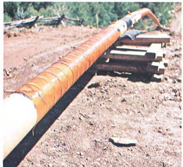
The pipe is wrapped to protect it from corrosion.
