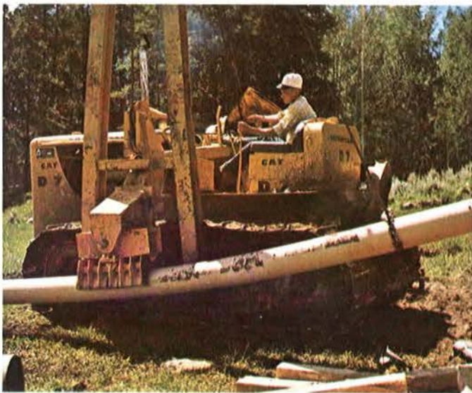
Pipe bending to meet horizontal and vertical alignment changes was used extensively on this job. In this way construction scars were held to a minimum and rehabilitation was made much easier.
