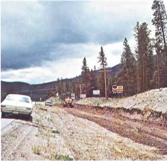
To eliminate additional scars on the landscape, existing rights-of-way such as this roadside were used to install the gasline.
