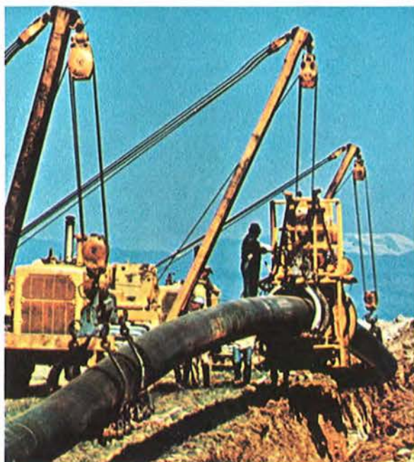
This machine is tape-coating a 24" pipe.
