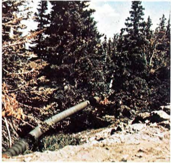
In one area of extremely erodible soils, the gasline was installed aboveground. Here it was wrapped and painted green to blend with the alpine trees.
