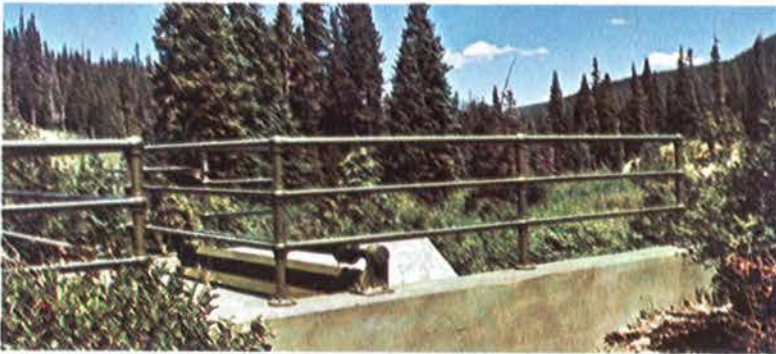
These objects were carefully colored to blend with their surroundings. The picture at lower left shows a utilities structure in the sunlight; the picture at lower right shows the same object in the shade.
