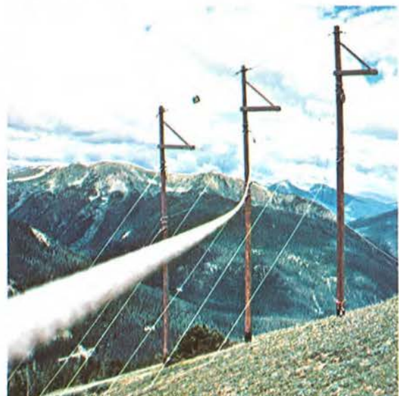
After the crossarms (if any) and permanent guys were attached, the nonspecular conductor was "pulled" by the tension-stringing method. The length of a "pull" depends on the situation—on this project, pulls ranged up to 5 miles in length.
