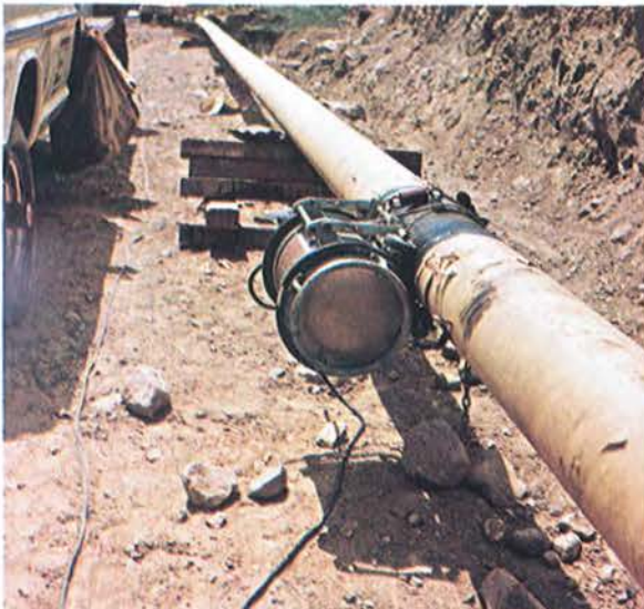
A portable X-ray machine checks the welded joint.
