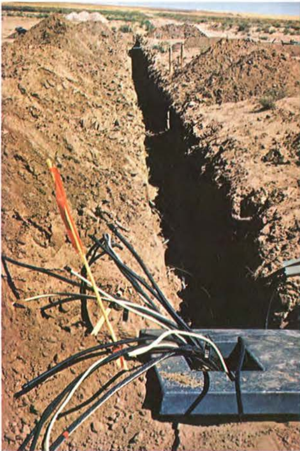
This concrete transformer pad is at the end of a distribution trench.
