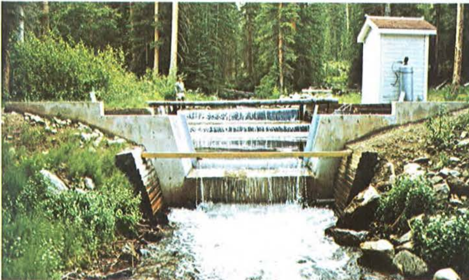
At weirs, water volume, temperature, velocity, and turbidity, are measured.
